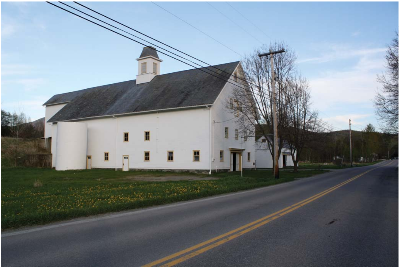
HC-1: Coming in to Huntington Center from the north. Jubilee Farm barn on the left.
