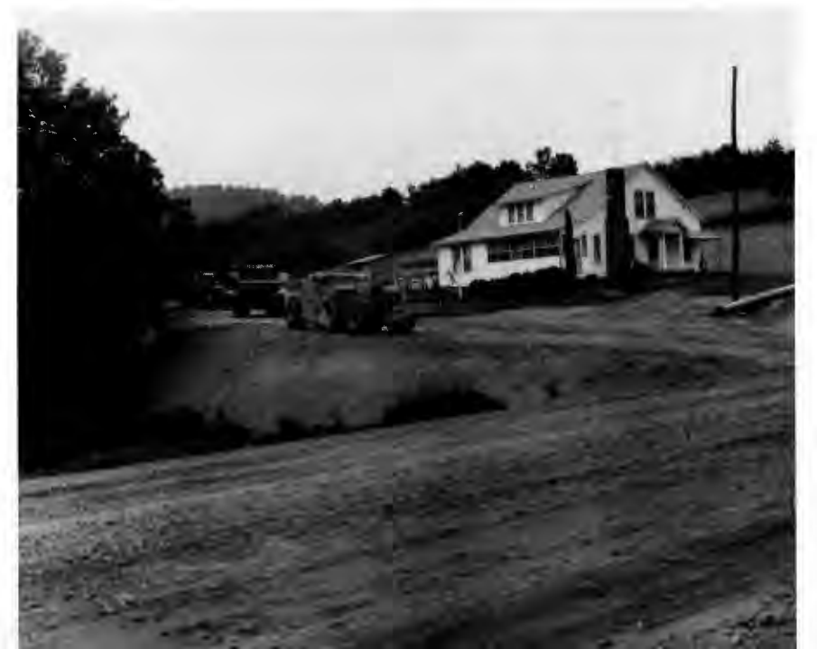
88. Cut-and-fill highway construction in the act of encouraging future spotty development: North Carolina Highway 19-E, between Spruce Pine and Crabtree, 1972. Surplus dirt from huge cuts is dumped as close to the cut as possible, setting up sites for future buildings.
