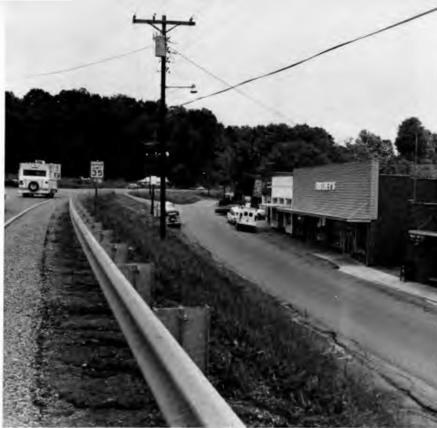
83. What is left behind after a major highway cutting is a two-level town such as Elk Park, North Carolina. The old stores, post office, etc., were strung out along an early road, right, until highway was cut into hillside. What you see here are Strips I, II, and III in one view.
