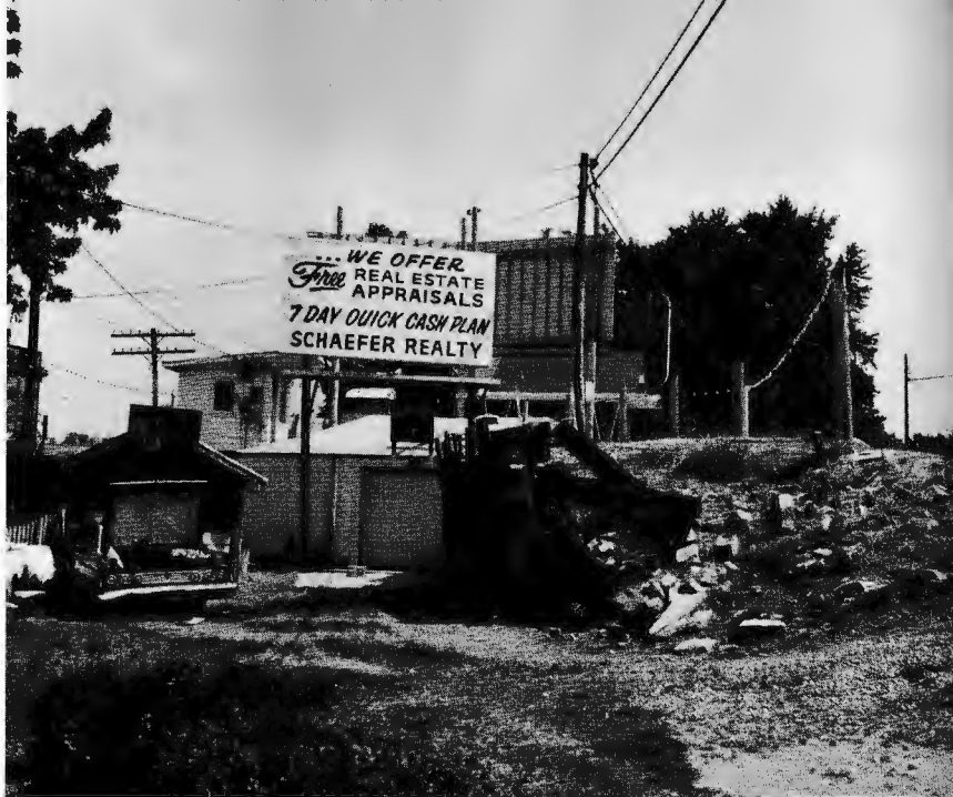
86. Early paved-road remnants show (bottom right), while later Dixie Highway (upper right) was built on earth fill to raise it out of the flood plain of the Driftwood and White rivers. Clear case of downgrading properties along older strip: note half-buried garage. Southern Indiana.
